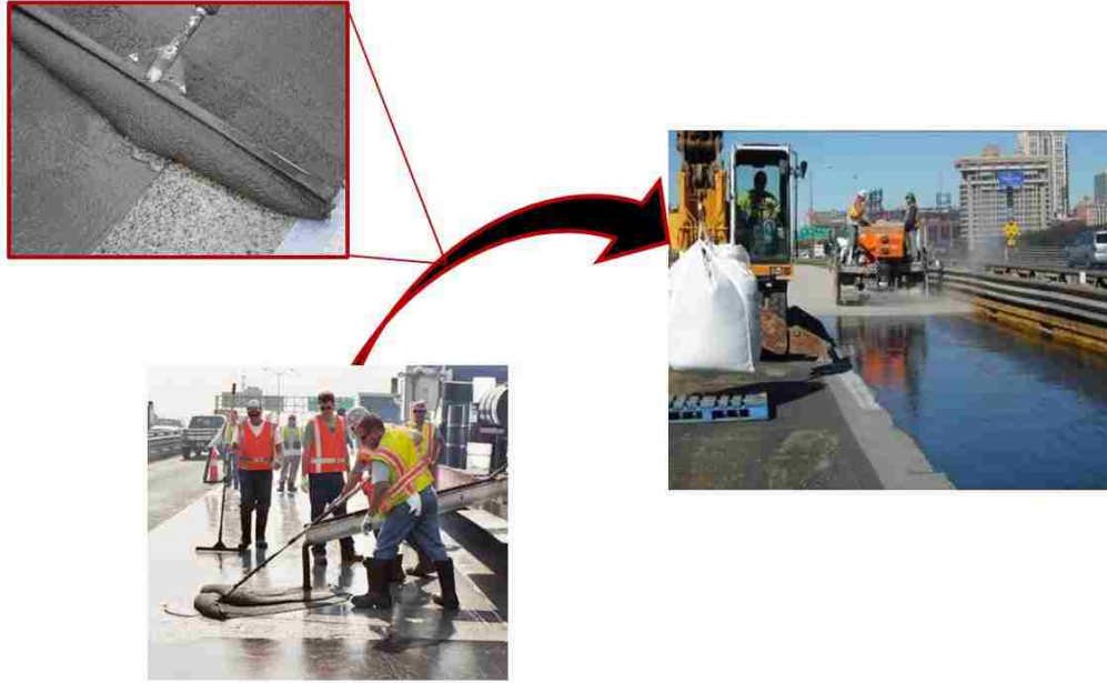
Figure 2.6: PC overlays in-situ courtesy of Transpo Inc.
